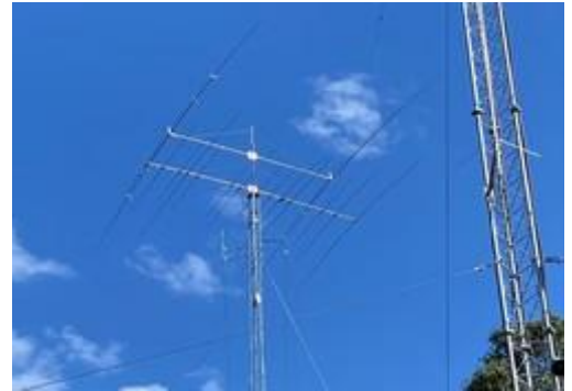
Tower 1 of the Tampa Amateur Radio Club, with the Force 12 C31XR antenna, second from the top. [Lu Romero, W4LT, photo.]
