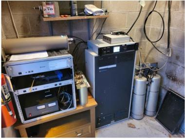
The 2 meter 'cans' are to the right. The test DR1X repeater is sitting on top of the old Motorola Micor repeater. On top of the DR1X is the filter for the input and the circulator for the output.
